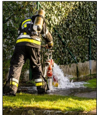
Image 1 A firefighter mounts a standpipe. (Picture: Pierre-Henri Demeyere)
