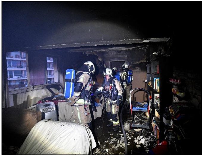
Image 11 View at the living room of the apartment. There is a lot of smoke damage in this room but nothing really burnt here. The fire was in the bedroom, where two firefighters are heading in the back of the picture. (Picture: Robert Decock)
