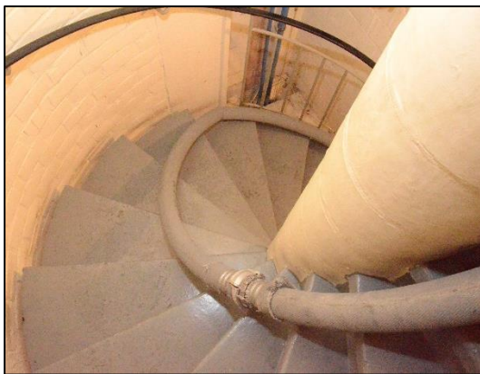
Image 7 View at the spiral staircase with the mobile riser hose on it. (Picture: Luc Van Ussel)
