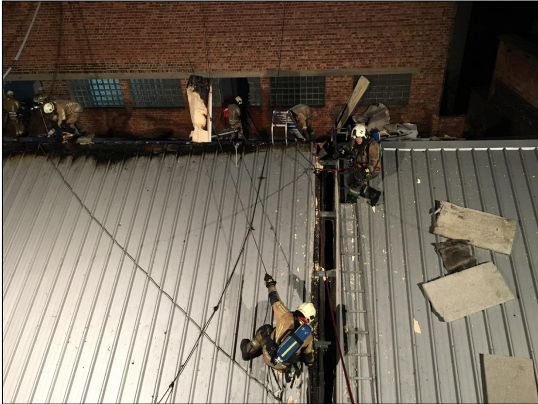
Image 12 As time passed, a trench was realized. On one side of the roof a cut was made along the full length. Because of this, the fire could not move further on that side of the roof. (Picture: Nicolas Freuville)
