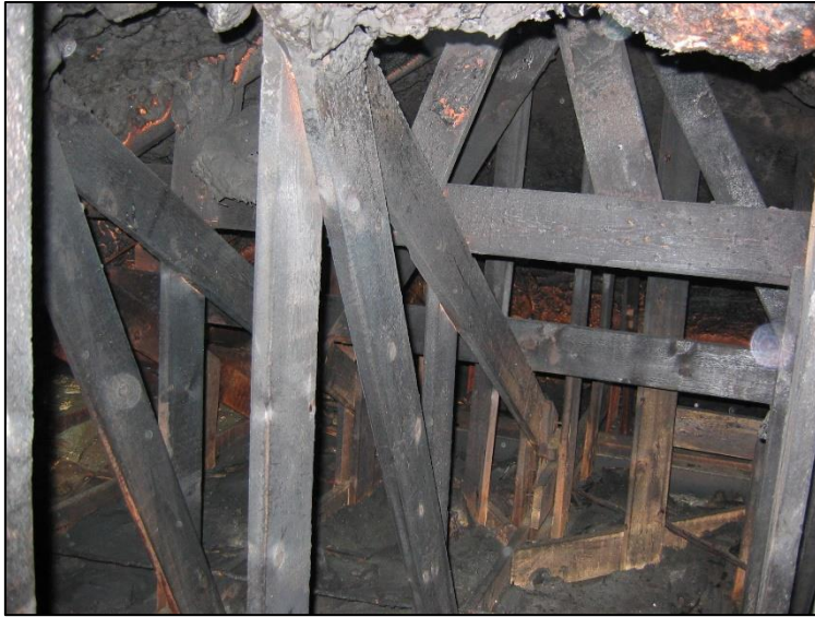
Image 2 The wooden support structure on the attic. The space between the rafters was rather limited. Because of this, the liberty of moving for the firefighters carrying SCBA was limited as well. (Picture: Diksmuide Fire Department)
