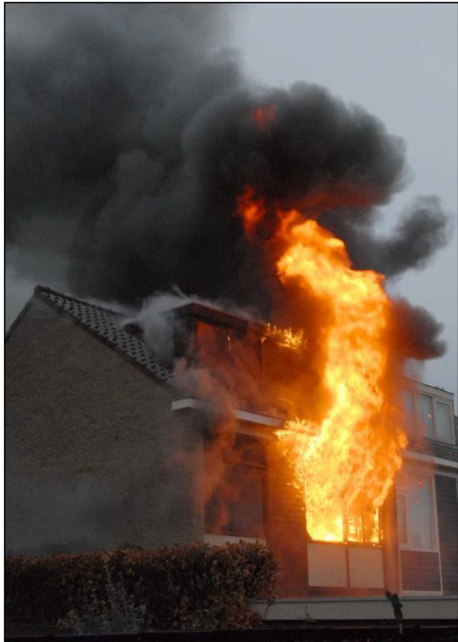
figure 3 A view of a fully developed fire venting out of two windows. (Photo: www.nufoto.nl )
