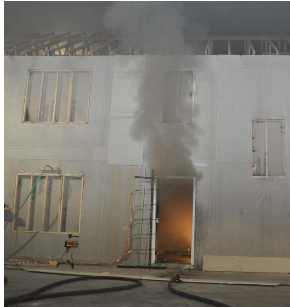
Fig 2.1 Smoke gas is exiting through the top end of the doorway while the rest of the doorway is being used for the supply of fresh air. This fresh air will allow for a rapid growth of the fire. (Photo: Steve Kerber – Underwriters Laboratories)
