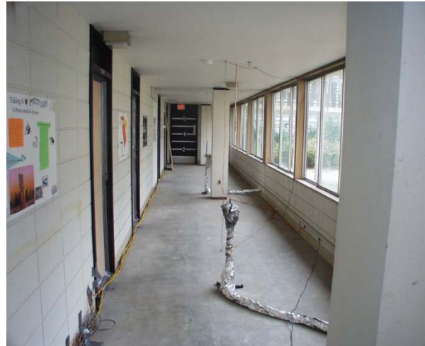
Fig 4.1 View on the hallway (Picture: NIST)
