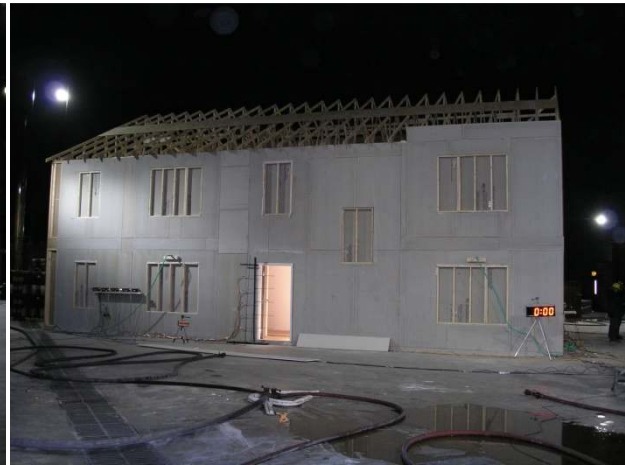
Fig 2.2 Two story house (297 m 2 ) (Photo: UL)
