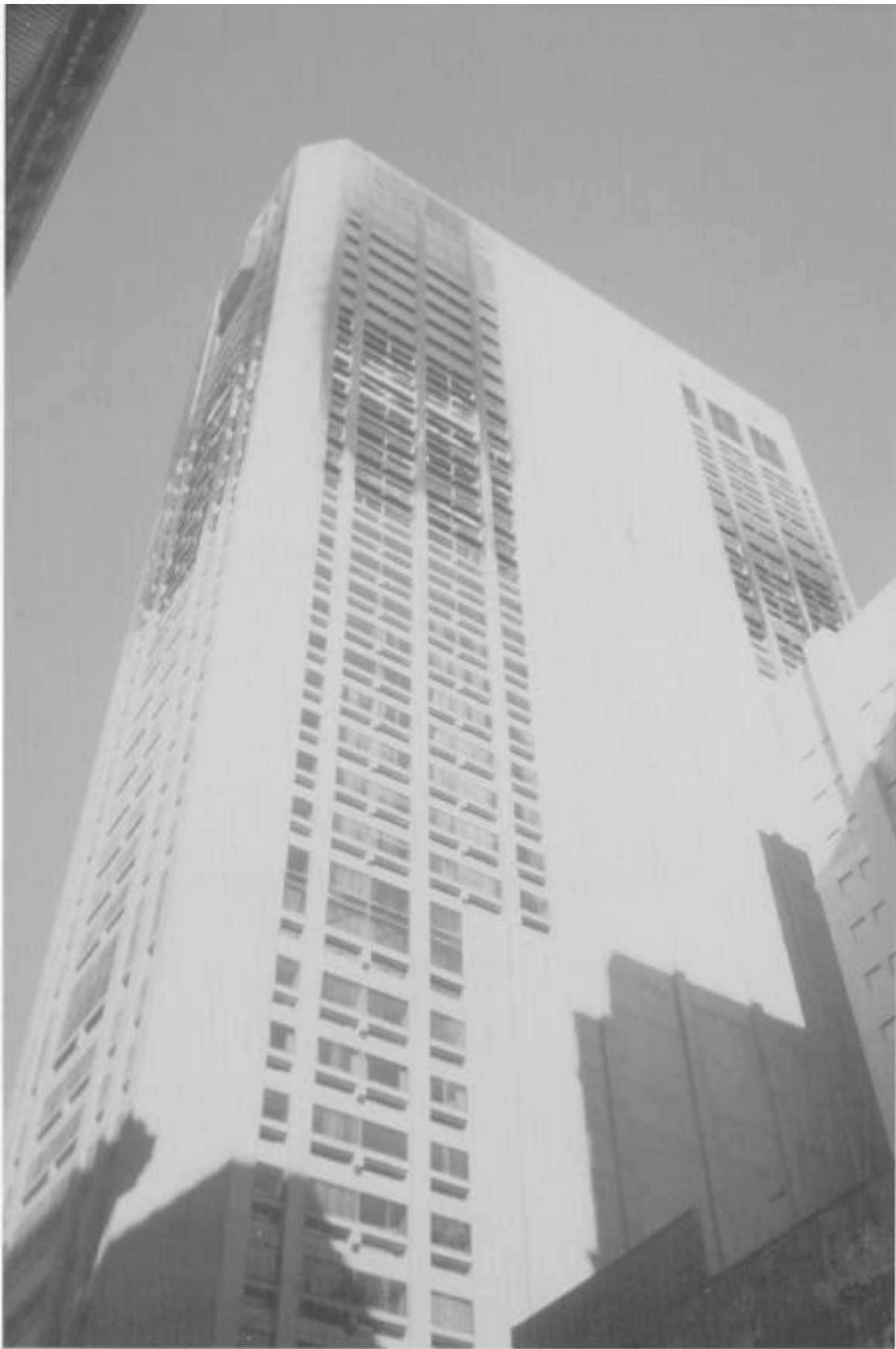
Exterior view of south side of building.
