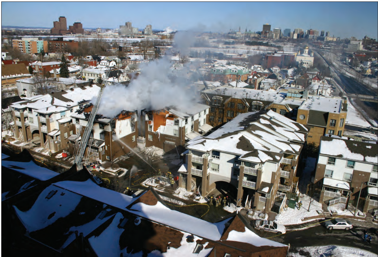
Photo courtesy of Ottawa Fire Services
