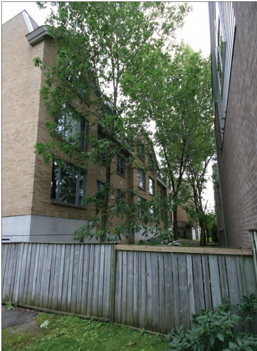
Rear of 202 Hinchey Avenue
