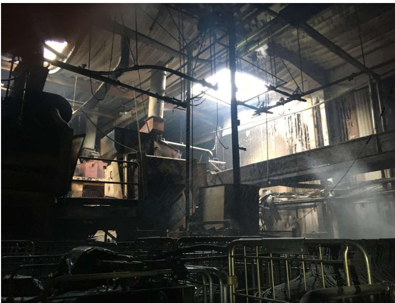
Figuur 18 Openingen in dak
