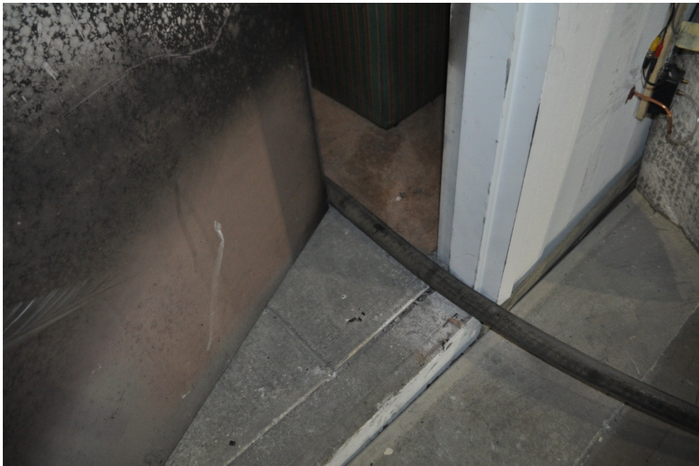
Figure 4.2: Door Control with a 1 3/4 inch Hoseline
