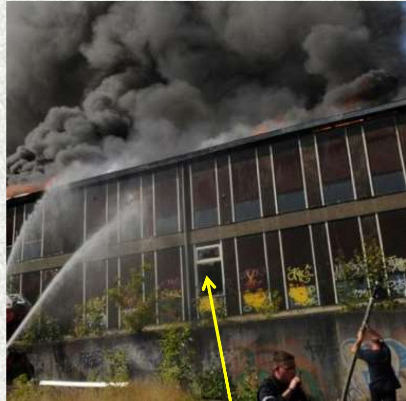
Entry to building made by squatters
